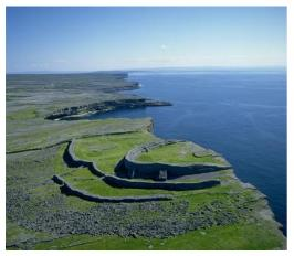
Dún Aonghasa (Inishmore, Co. Galway) was built on a clifftop, giving it defensive advantages over any attacking from the sea. There are 3 dry-stone walls (meaning without mortar) encircling the fort. In addition, some of the areas between the walls are filled with jagged blocks of stone, (a
